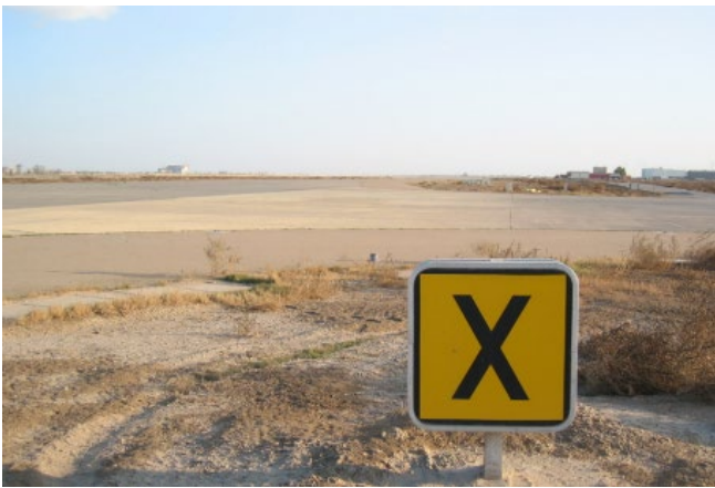
Fig 2. Use "X" for Closed Taxiway Marker
