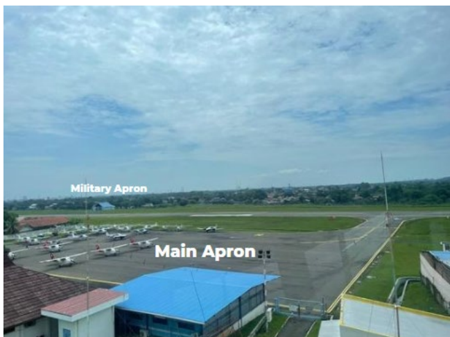
Fig 1. The location of the Military Apron and Main Apron from the Tower
