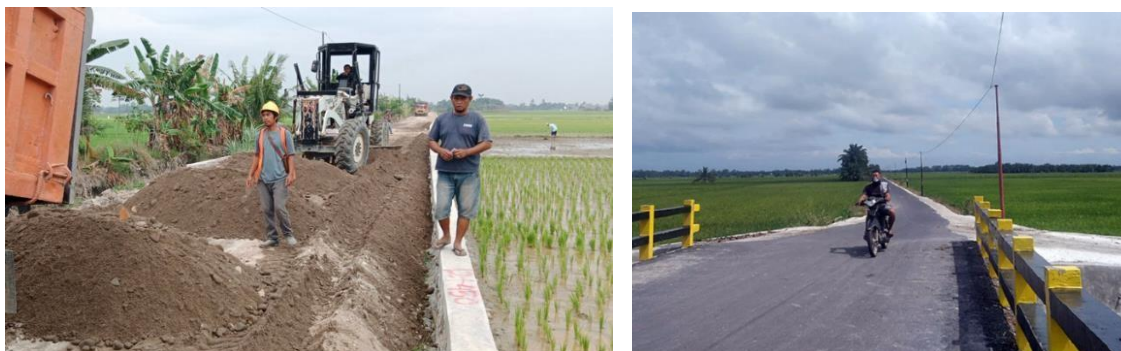
Figure 1.1 Road infrastructure in Rawang Panca Arga, Asahan Regency
